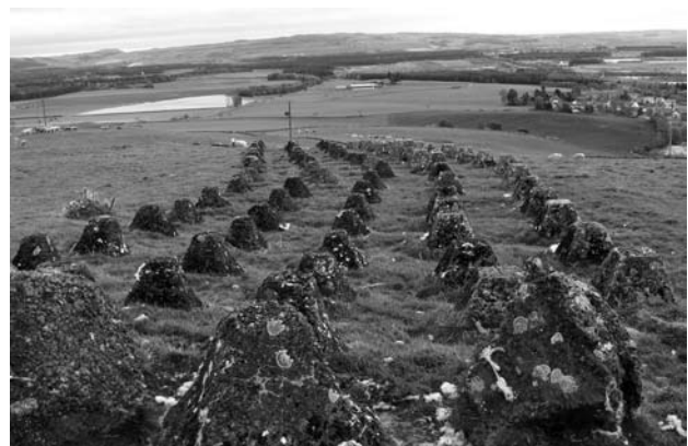
Illus 26 To the north of Collessie a well-preserved section of 'pimples' provides the A/Tk barrier over an area of bedrock, between sections of A/Tk ditch. The two rearmost rows (right) are larger.
