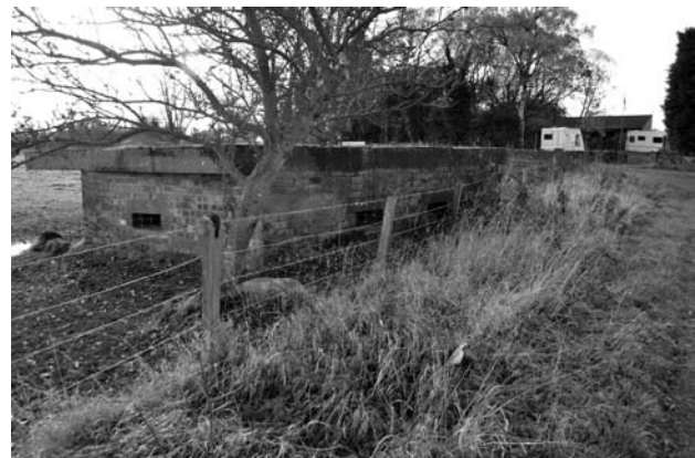
Illus 6 The north-facing wall of the HILLMAN pillbox showing the Bren Gun and A/Tk Rifle embrasures.
