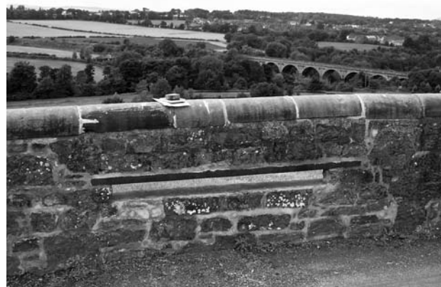
Illus 14 Firing position in the southern wall of St Drostan's Cemetery, Markinch (location, Illus 13), the lintel formed by tram rail sections.
