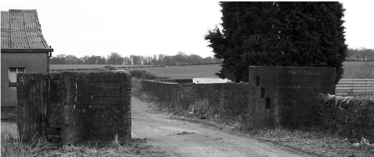
Illus 11 Road block RB69 at Cowdenlaws Farm (location, Illus 10 ), with part of the 43m-long A/Tk wall visible behind. This type of road block relies on three sections of tram rail inserted into vertical slots or horizontal wood-lined sockets.
