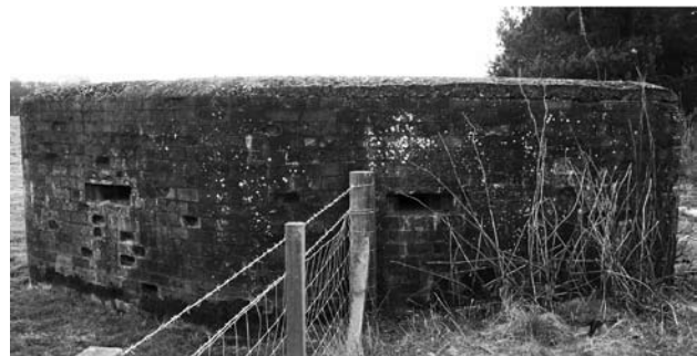
Illus 7 The SWEETHOPE pillbox (serial number South 11; Illus 17, a Type 24 Bren Gun pillbox, immediately beside the main railway line just NE of Ladybank junction, covering the blocks on the railway (Illus 21).
