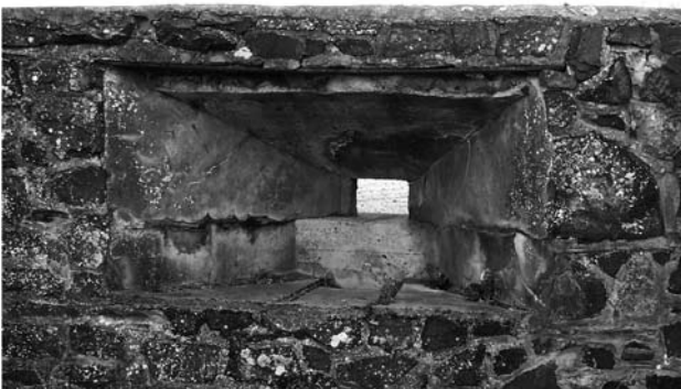
Illus 20 A pre-cast loophole of the same kind as is used in many of the pillboxes is set into the SE corner of the garden wall at Loanfoot, close to the pillbox with the same name.
