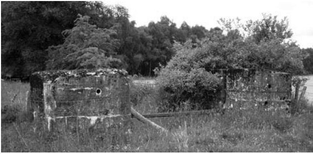
Illus 44 Road block RB131. In this type of horizontal rail block the three rails are rested on steps within a single vertical slot. The holes on the eastern side are formed by pipes around which the concrete was cast – their purpose is not known.
