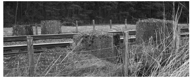
Illus 21 Concrete A/Tk cubes flanking the location of Rail Block E on the Edinburgh–Dundee main line (Illus 17).
