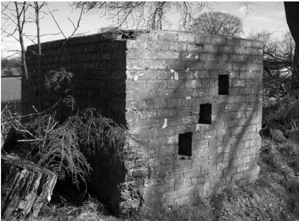
Illus 19 One side of the horizontal rail block RB78, surviving on a farm track. The block is made of concrete poured into brick shuttering.
