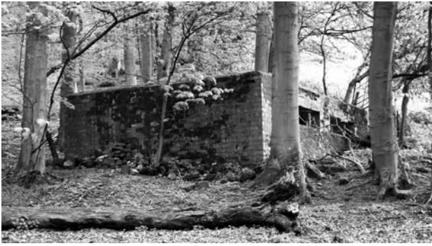
Illus 31 The rectangular double-embrasure medium machine-gun pillbox in KINFAUNS WOOD (serial number North 2; Illus 30), overlooking the blocks on the main Perth to Dundee road and railway.
