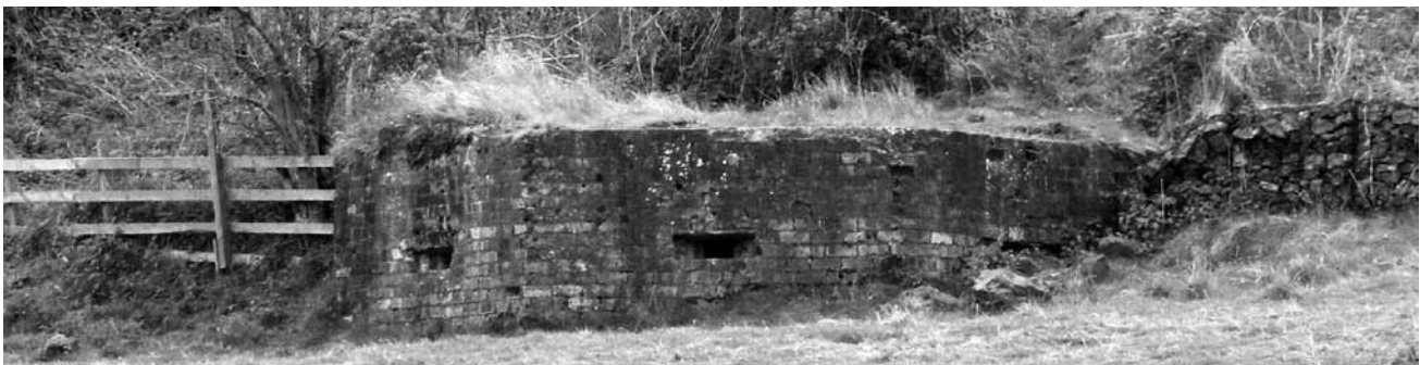
Illus 29 The FORT pillbox near Newburgh (serial number South 15; Illus 28) partly buried under slip from the railway embankment behind it.
