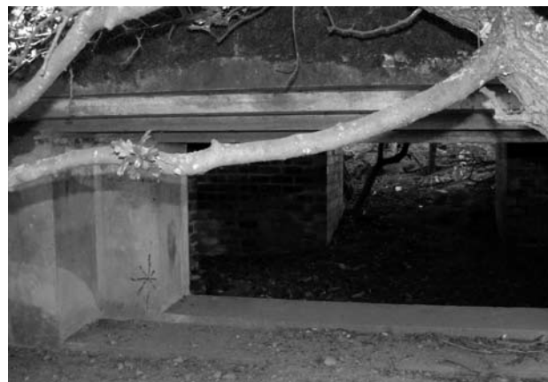
Illus 36 The embrasure of the Circles A/Tk gun chamber, remaining traces of camouflage paint on the concrete. The aperture through which the gun would be wheeled from the rear is visible.
