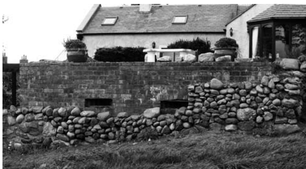
Illus 25 The CASK HILL pillbox (serial number South 13; Illus 24), set on the edge of Collessie village and faced with stone on the south side to disguise it as part of the field wall. This is one of the Command Line variant Type 24 pillboxes, where there are two loopholes on one wall to accommodate a Bren Gun and Boys A/Tk rifle side by side.
