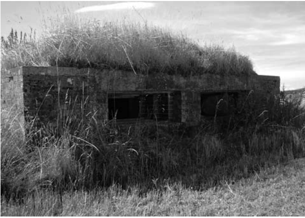
Illus 8 The STARVIEW pillbox (serial number South 4). This type (without a type number) resembles a design erected by the British Expeditionary Force in France (Osborne 2008, 155–6) and is found in the UK only on the Command Line. It was intended to house a pair of Vickers medium machine guns.
