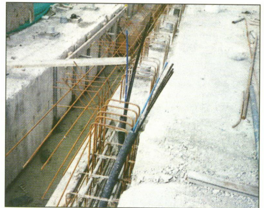
Figure 12: Spreader Beam construction on the Dock Quays.
