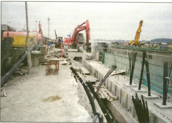
Figure 9: Subway roof demolition
