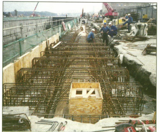
Figure 13: Subway Roof Reconstruction following Anchor Stressing
