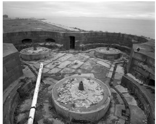
Illus 8 The trefoil arrangement of gun platforms on the summit of the Leith Martello Tower.
