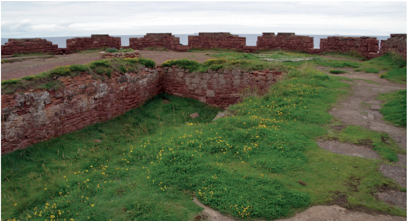
Illus 5 The interior of Dunbar Battery as it survives (R Morris)
