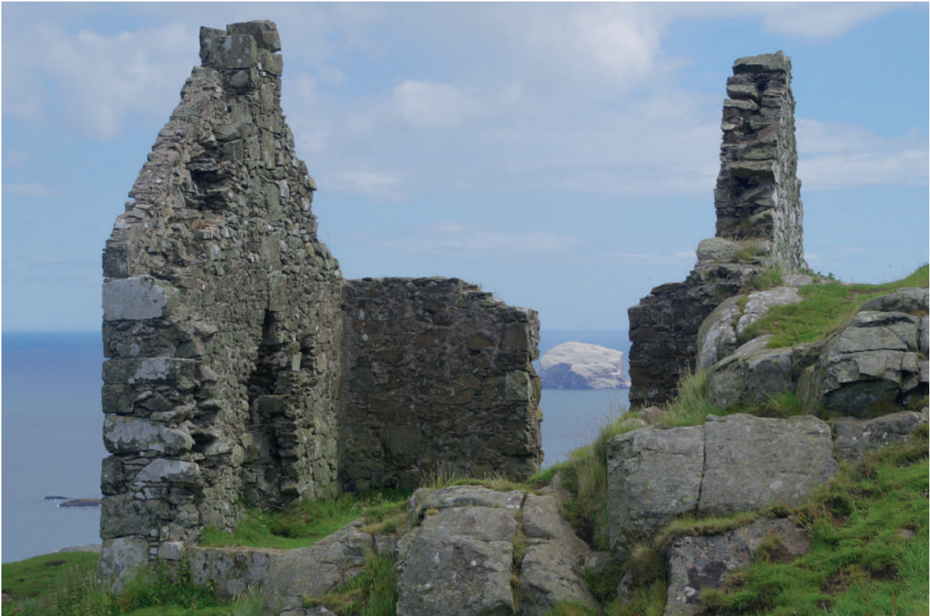
Illus 2 The accommodation hut for the Signal Station on the summit of North Berwick Law. (R Morris)
