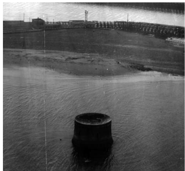
Illus 7 The Martello Tower, photographed from the air in 1951. (Reproduced by permission of the National Collection of Aerial Photography ncap.org.uk NCAP-000-000224-823)
